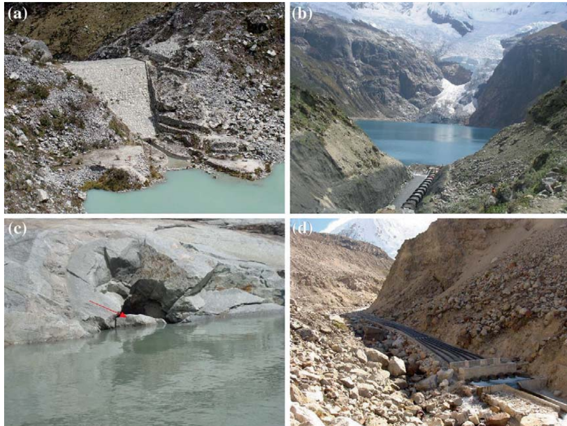
Fig. 9 Examples of remedial works. Part a shows artificial dam and concrete outlet of lake Llaca in the central part of the Cordillera Blanca; dam freeboard is 12 m. Part b captures ongoing work on the dam of lake Rajucolta in 2004. Part c shows the entrance to the tunnel excavated in the bedrock dam of lake No. 513 ( red arrow ). Part d shows six siphons installed in fall 2011 to drain and lower the water level of lake Palcacocha
