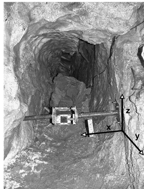
Fig. 10. The TM71 deformer installed across the monitored fissure in the cave Na Pomezí (site P1).
