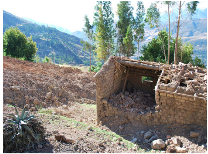
Fig. 10 Farm house destroyed by stones transported aerially ( h in Fig. 4). Accumulation with depth up to 1.8 m ( g in Fig. 4) can be seen left from the house
