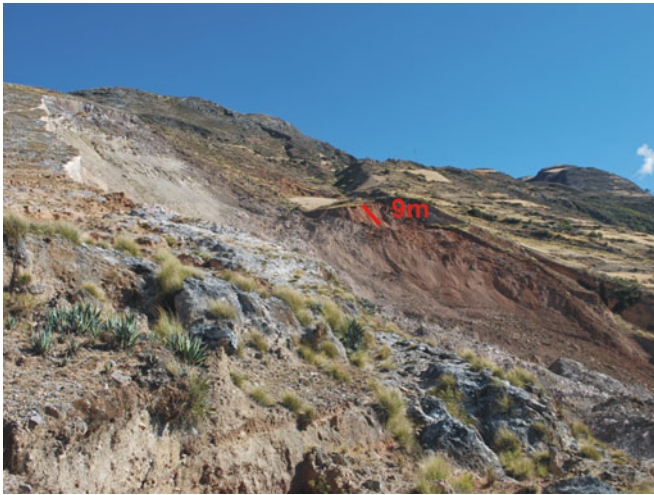
Fig. 8 General view of the main scarp and depletion zone of the landslide ( a , b , and c in Fig. 4) from east to west
