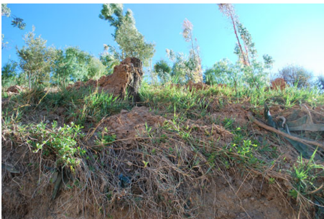
Fig. 9 Splashes of landslide material on stable ground ( g in Fig. 4) indicate that the material came from left to the right of the photo
