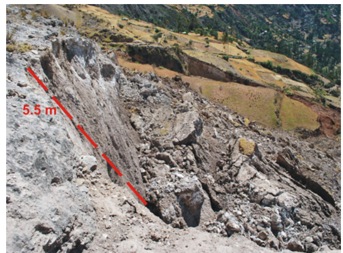
Fig. 7 Main scarp of the complex landslide ( a in Fig. 4) with well visible minor scarps with opened cracks and rock blocks with slightly back-tilted surfaces
