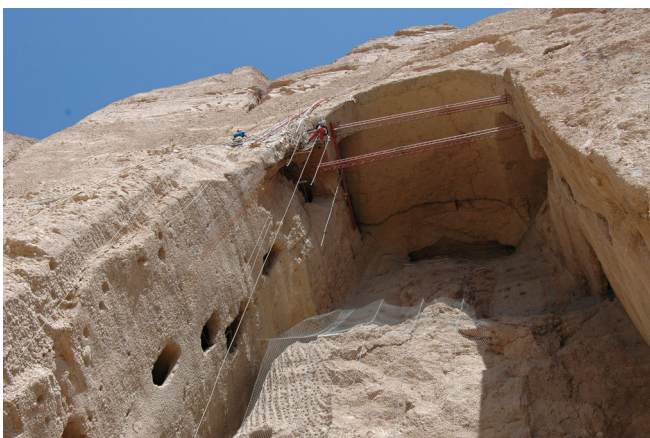
Fig. 5 Climbers at work on stabilization of the left side of the Eastern Giant Buddha niche
