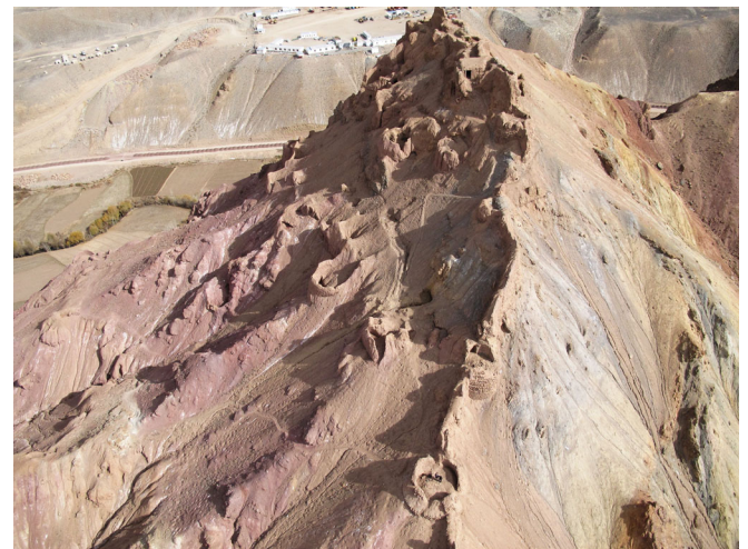
Fig. 6 The upper part of the Shar-e-Zohak red fortress. Damage to buildings and archaeological remains is quite evident. Aerial photo from drone (Courtesy of Iconem)
