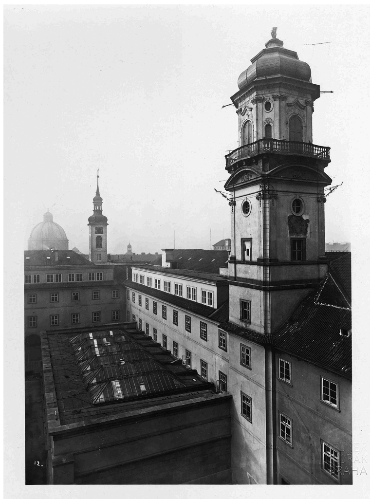
Fig. 1 Clementinum astronomic tower in the 1930's. Source: Archives of the National Library of the Czech Republic
