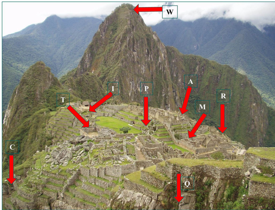
Fig. 1 Location of the dilatometric measurements (view to the N with Waynapicchu Mt. in the background). The flat central part of the Machupicchu site represents the main square between points T and P. The inset shows manual measurements with a rod dilatometer. C = Cave, T = Principal Temple, I = Intiwatana, P = Plaza, W = Waynapicchu, A = Acllawasi, M = Mirador, R = Rodadero, Q = Qhata
